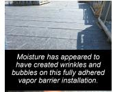
The finish of your concrete roof is important and depends on your roofing and or vapor barrier system...
